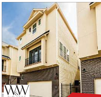
5525 Petty Unit B Cottage Grove
