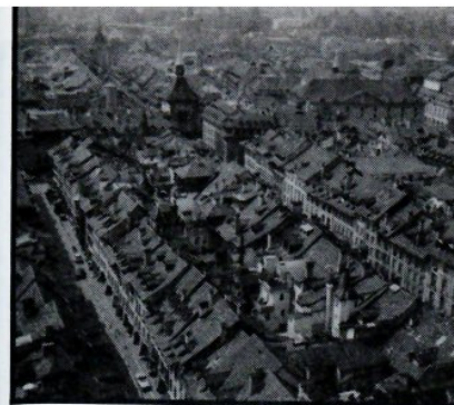
View of old-town Bern with its irregular roofs.
